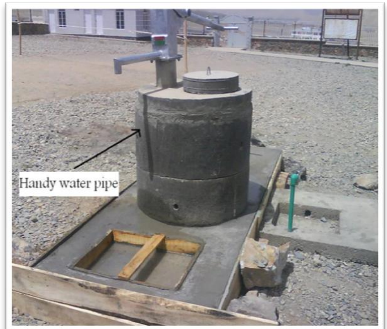
Our new hand water pump built by the local PRT
